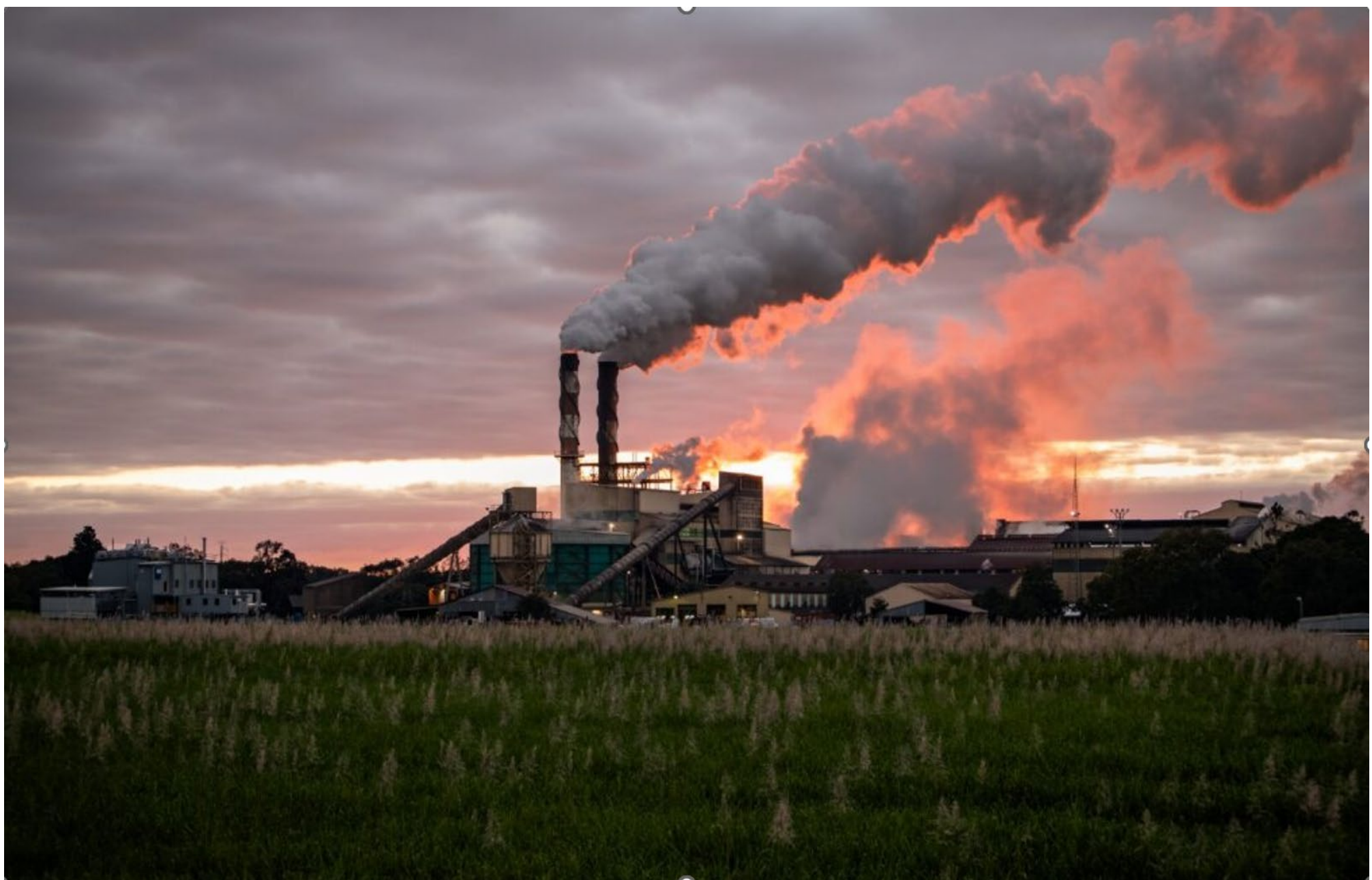
Mackay's Racecourse Sugar Mill, which houses the QUT Pioneer BioPilot Plant Picture must be credited to Queensland University of Technology if used.
